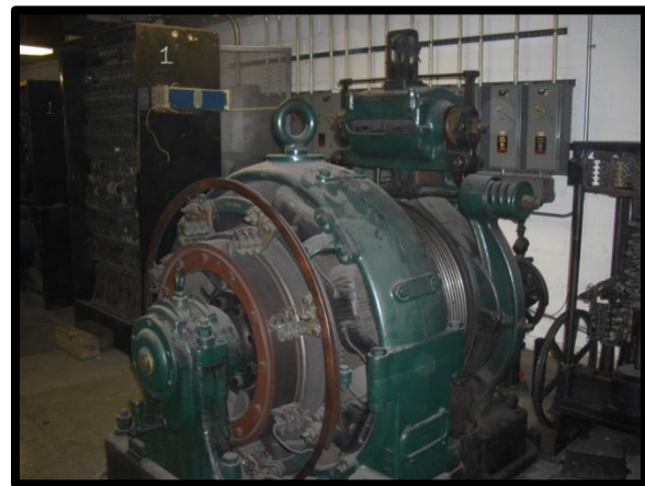
Figure 6: Original Elevator Motors
