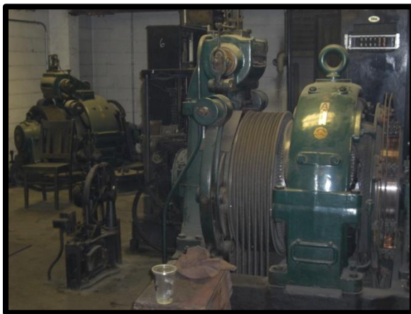
Figure 5: Original Elevator Motors
